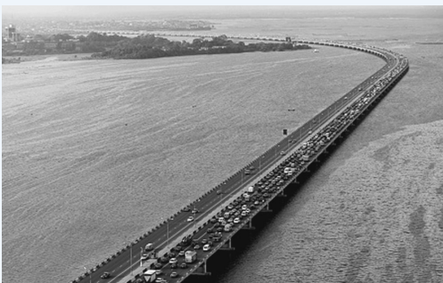
Third mainland bridge
